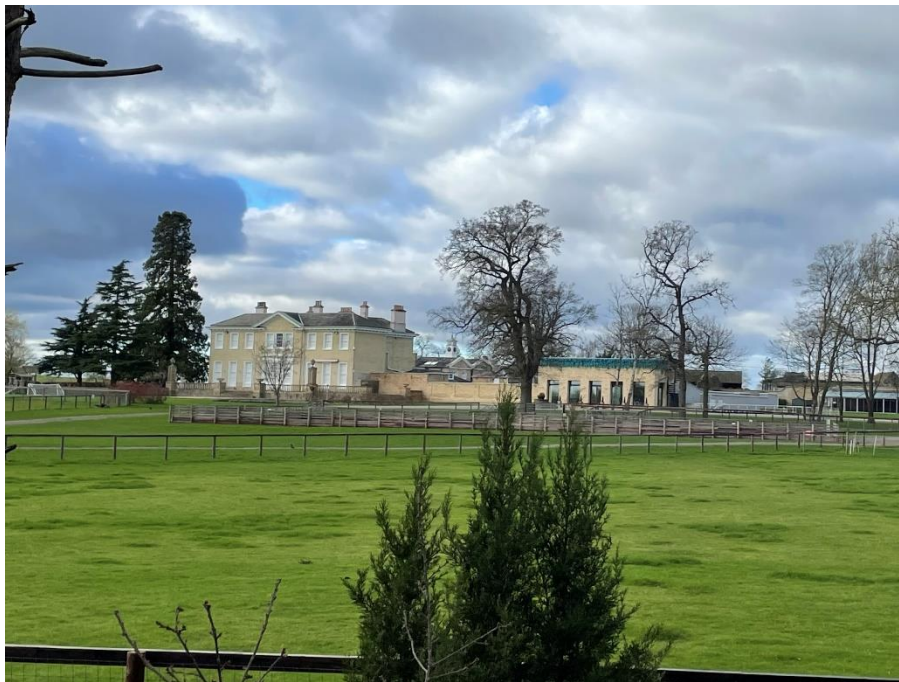
Plate 31: As-built pool house when seen from the Grade II Listed Cricket Pavilion.
